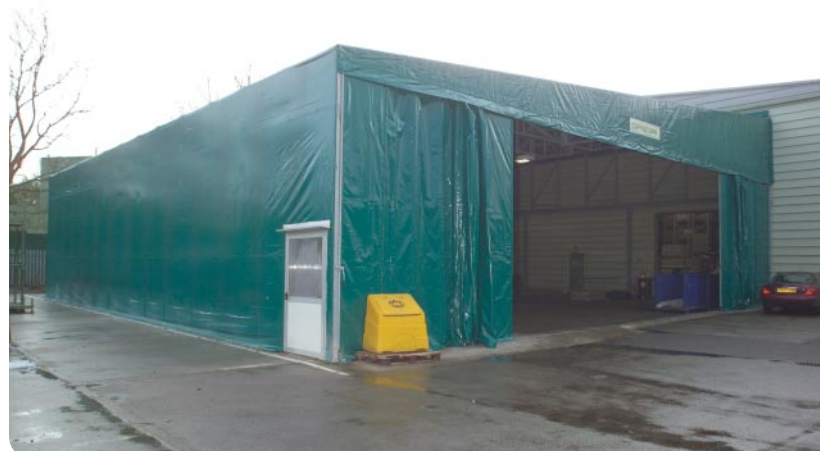
Landsdon has recently installed its second CopriSystems canopy.
